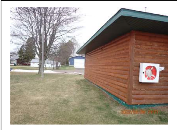
21. Gile Park – Restrooms (2)
