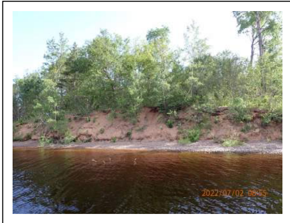
19. Island #5 – Bank erosion
